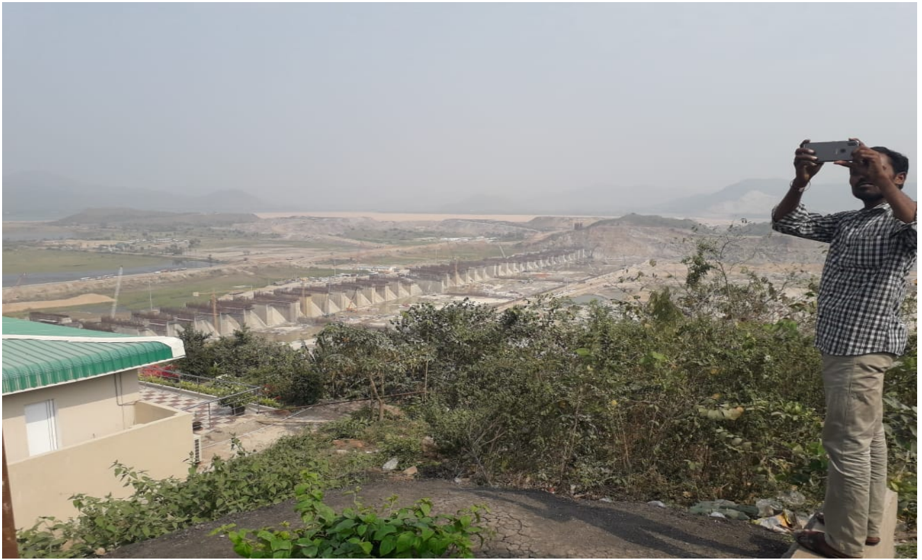
Polavaram Project Hill View
